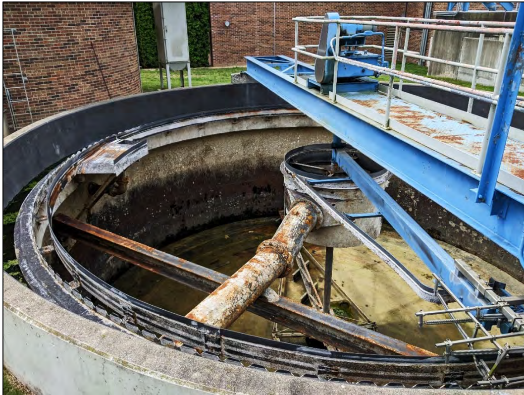
Figure 6 – Final Clarifier #1, Dewatered for Inspection
