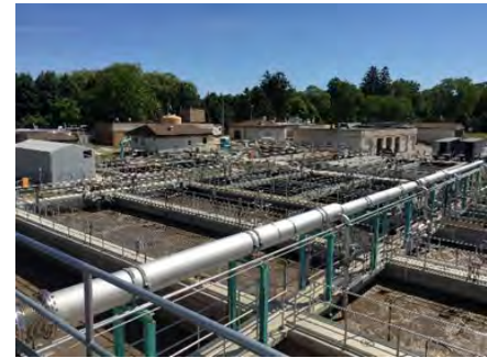
Completed Plant with Aeration Tanks
