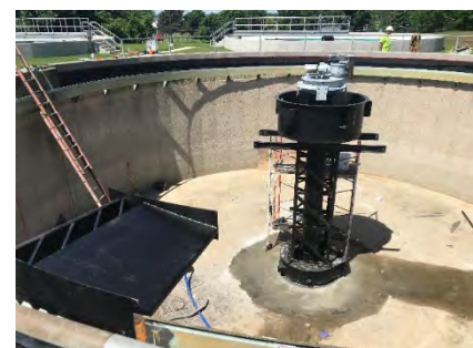
Replaced Final #3 Mechanism & Internals
