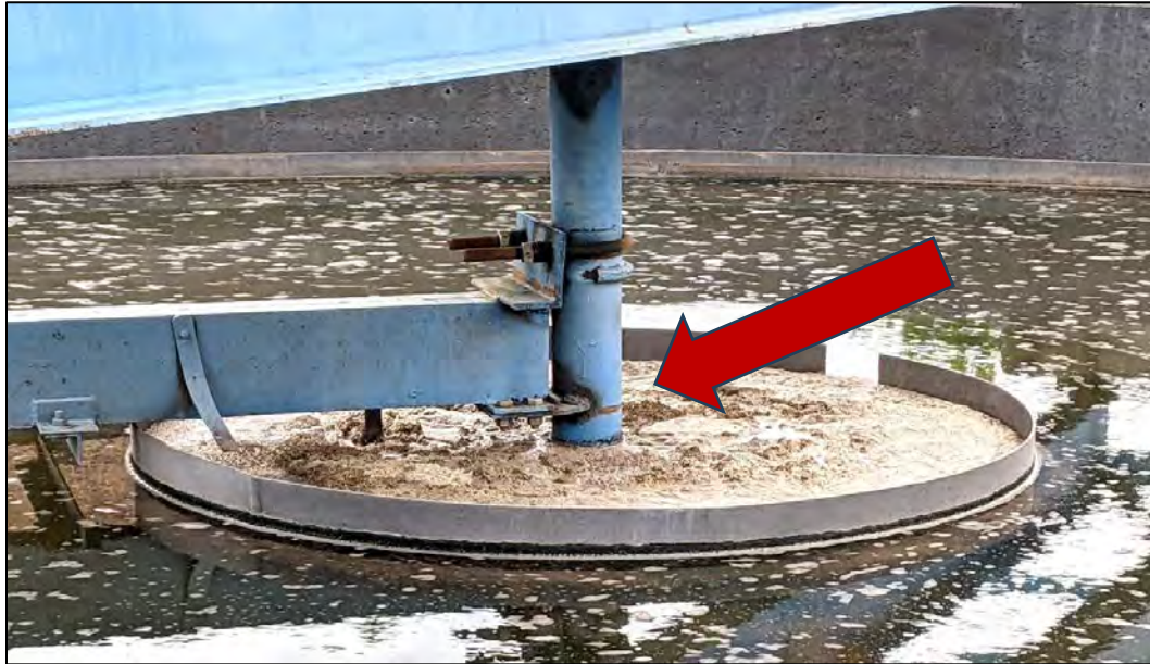
Figure 2 – Drive Tube for Final Clarifier #2 (showing location of repair)
