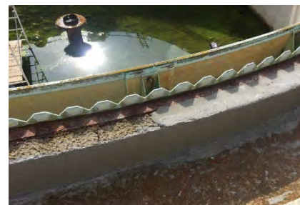
Concrete Trough Repairs in Progress
