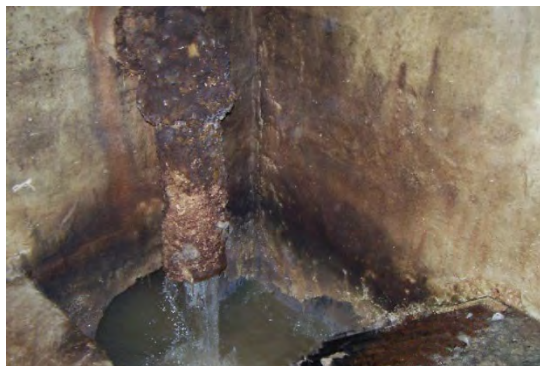
Old Manual Bar Screen in Confined Space is Now Replaced by Picture to the Right
