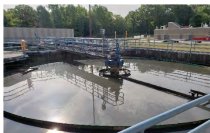
Repair of "Square" Final Clarifier, SCCMUA WWTP
