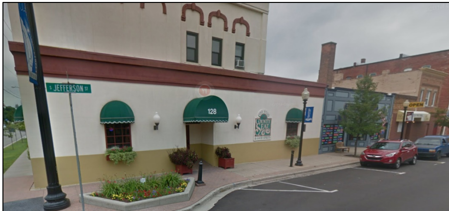
Jefferson Street Frontage (east elevation)
